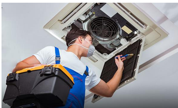
Air Conditioning FCU Preventative Maintenance
